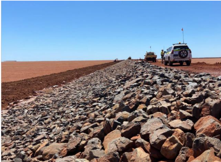
NORTHERN EMBANKMENT TRIAL
