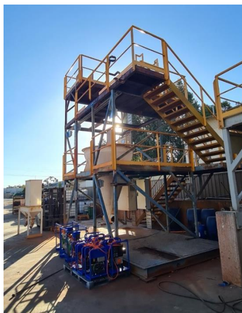
Figure 2: Salt Pilot Plant Under Construction
